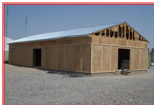
The Lumberjack Shack – almost completed!
