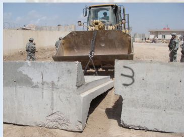
A 3 rd PLT Soldier uses a 5-yd Bucket Loader to move a barrier.
