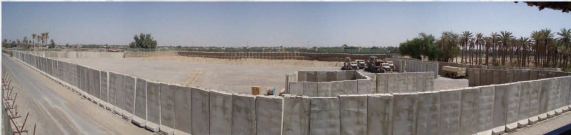
1 st Platoon Construction Mission at FOB Justice – After
