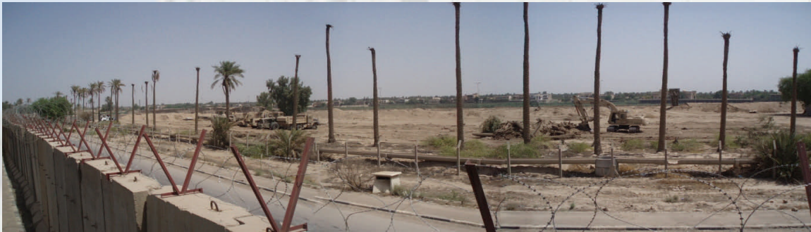
1 st Platoon Construction Mission at FOB Justice – Before
